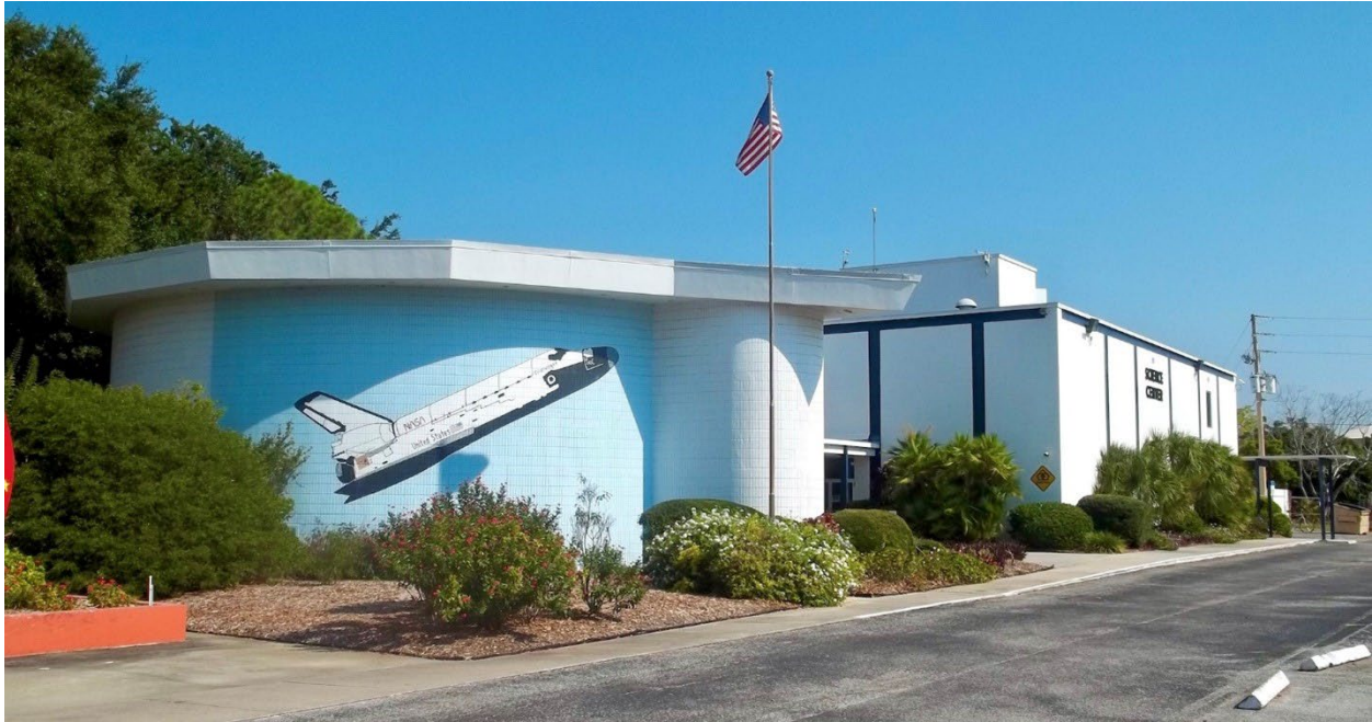
Figure 3-1. View from the parking lot of the circular wing (rotunda) and mural with rectangular wing in right of frame. The rectangular wing will be replaced by a triangular garden and triangular structure; these will occupy the same footprint as the existing structure.
