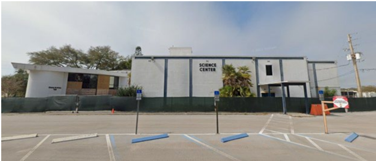
Figure 3-2. Google Street View of the current condition of the Science Center.
